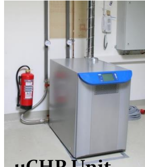
µCHP Unit (Gas to DC Grid)
